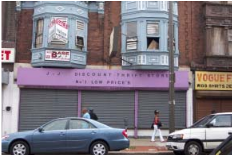
Deteriorated properties between Arch and Walnut will be renovated and re-tenanted
